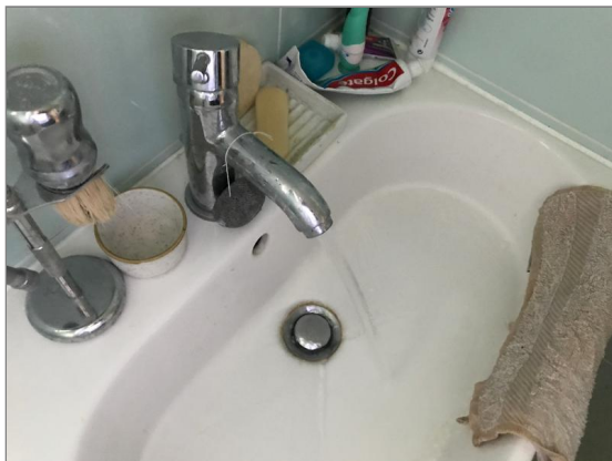
Photo - 112 Testing hot water supply with one outlet open.
