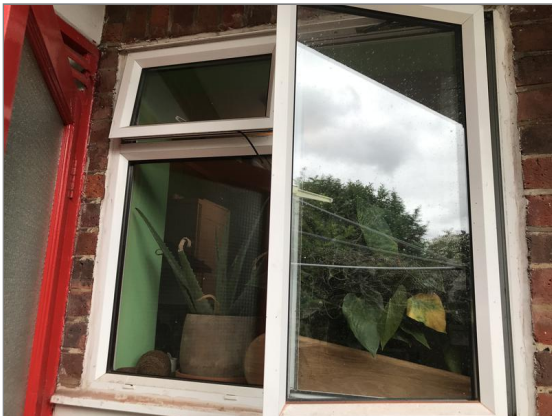
Photo - 16 Kitchen windows.
