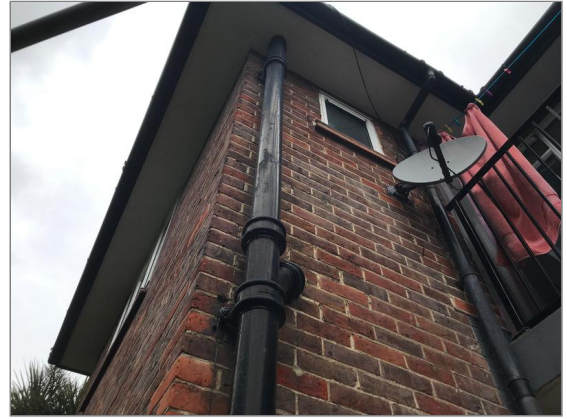
Photo - 115 Cast iron soil stack at rear of property.
