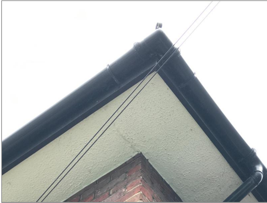
Photo - 29 Decorations applied to fascias and soffits around the property.
