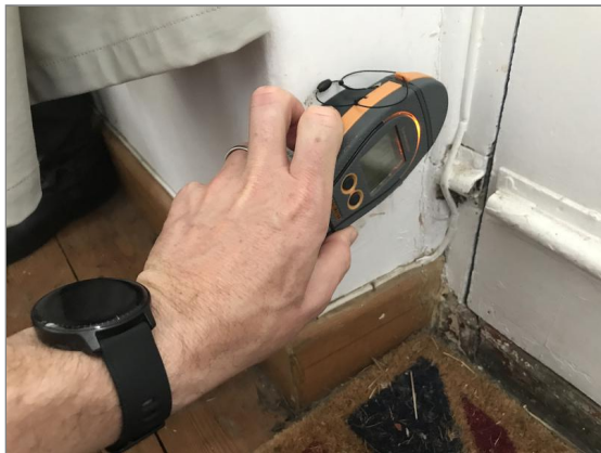
Photo - 43 Damp meter testing to entrance hallway.
