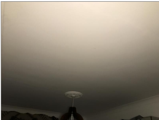
Photo - 36 Bedroom ceiling.
