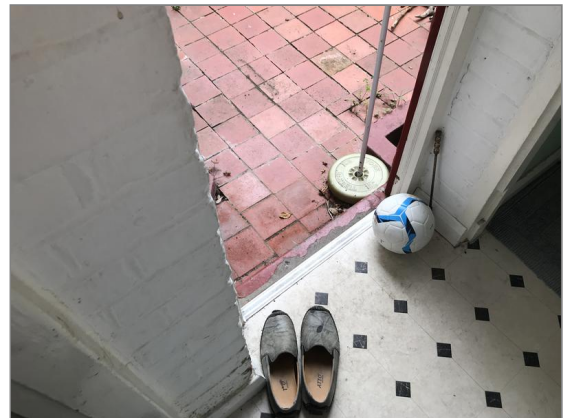
Photo - 62 Rear hallway walls.
