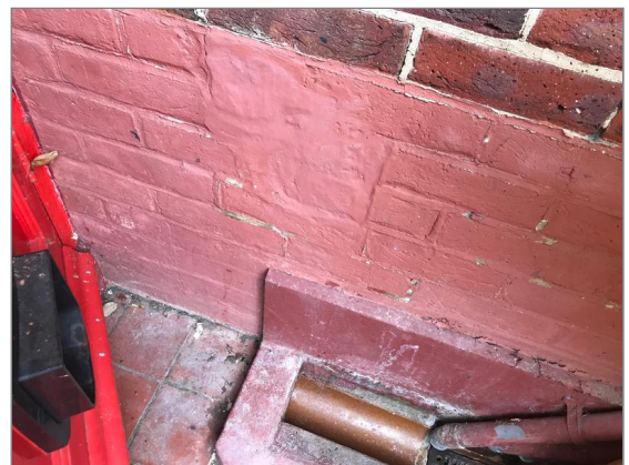
Photo - 64 Decorations applied to external finish walls.
