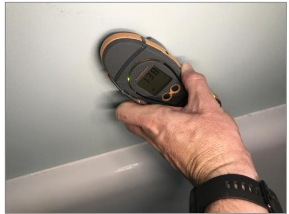
Photo - 60 Damp meter testing to bathroom walls.
