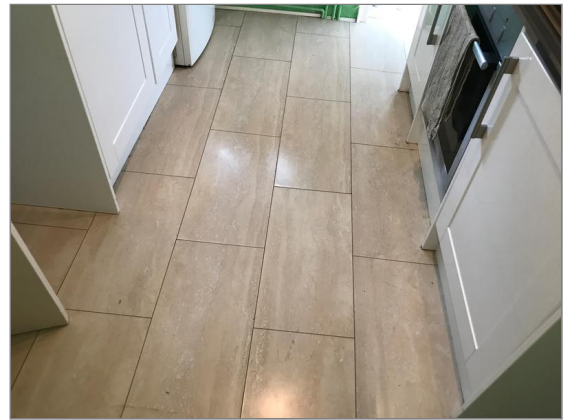
Photo - 69 Kitchen floor.
