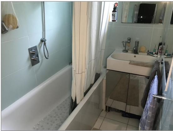
Photo - 59 Bathroom walls.
