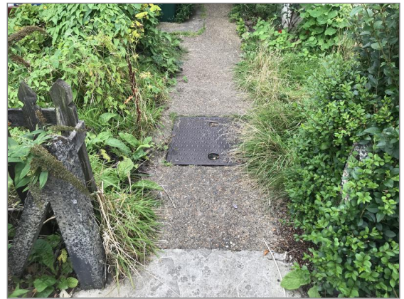
Photo - 119 Oversite concrete forming path in front garden.
