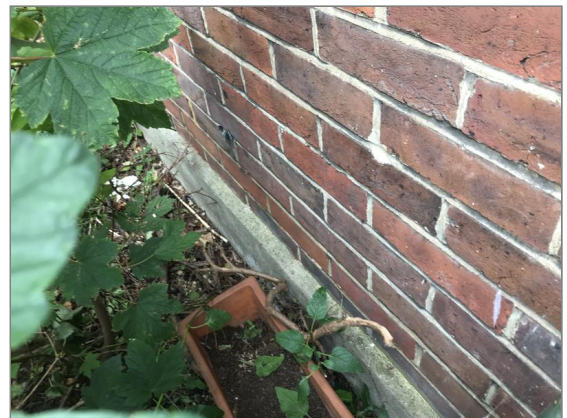
Photo - 13 Render applied to lower part of walls.
