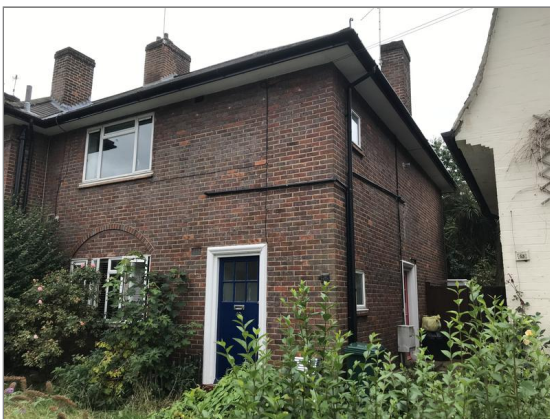
Photo - 9 Rainwater guttering running around main roof.
