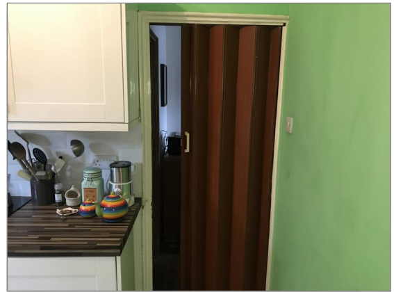
Photo - 93 Plastic concertina door leading to kitchen.
