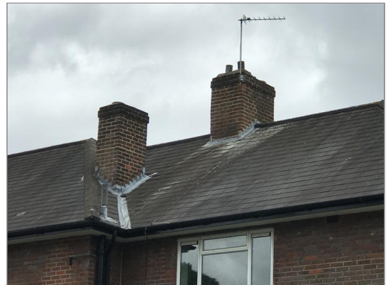
Photo - 5 Main chimney stack located above apex of roof.
