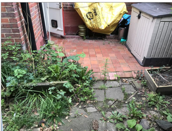
Photo - 128 Orange quarry tiles in rear garden.
