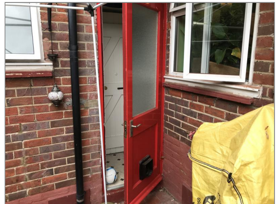
Photo - 26 Rear garden door.
