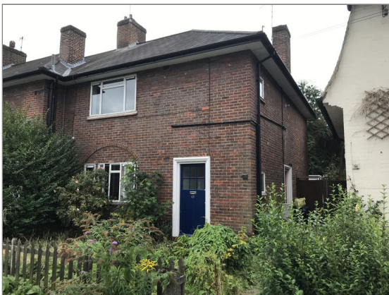
Photo - 12 External brickwork walls.
