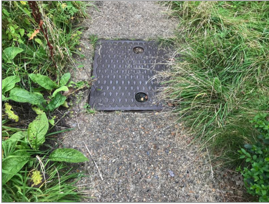
Photo - 114 Inspection chamber in front garden.
