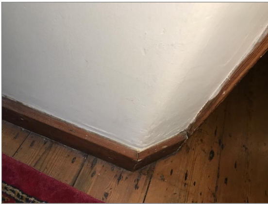
Photo - 92 Exposed timber architraves and skirtings.
