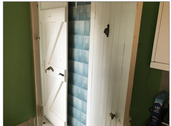
Photo - 95 Timber door at rear of dwelling.
