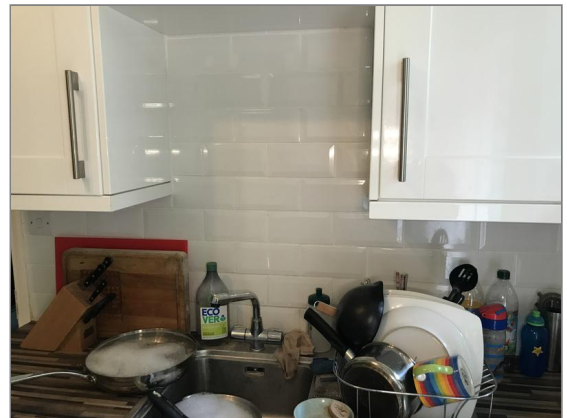
Photo - 56 Kitchen tiling.
