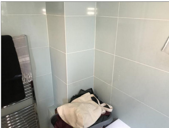
Photo - 61 Bathroom walls.
