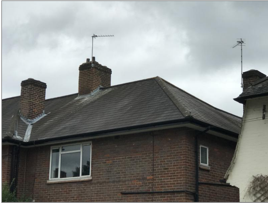
Photo - 7 Front pitched roof coverings.
