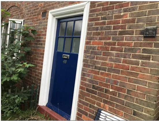
Photo - 23 Front door.
