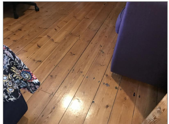
Photo - 77 Living room floor.
