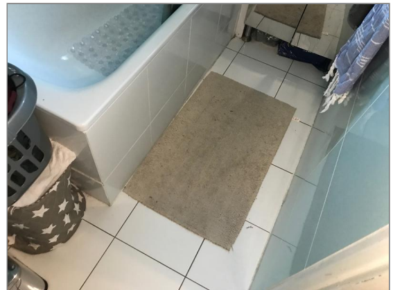
Photo - 71 Tiling in bathroom.
