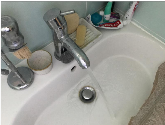
Photo - 106 Testing cold water supply with one outlet open.
