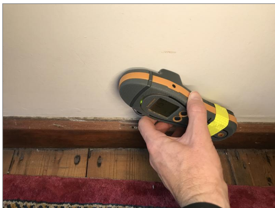
Photo - 45 Damp meter testing to entrance hallway.
