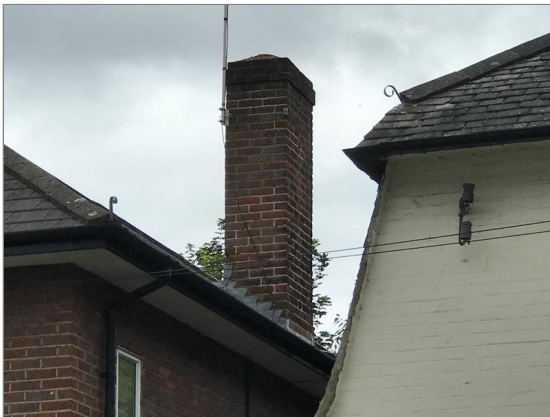
Photo - 4 Chimney stack located to right hand side of property.
