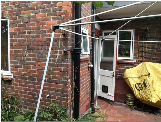
Photo - 14 Paint applied to rear walls.
