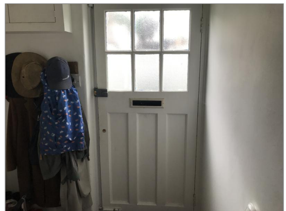
Photo - 28 Internal view of front door.
