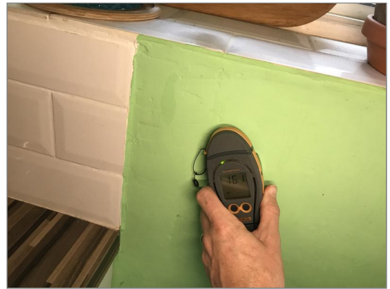
Photo - 54 Damp meter testing to kitchen walls.
