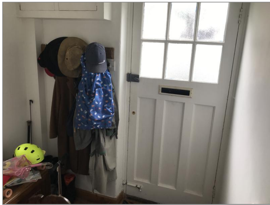
Photo - 41 Entrance hallway walls.
