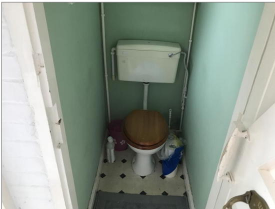
Photo - 65 WC walls.
