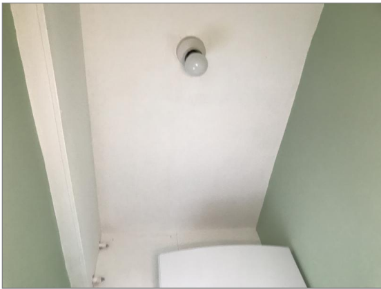
Photo - 40 WC ceiling.
