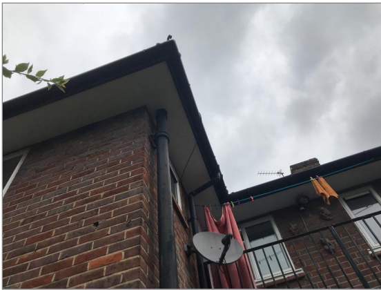
Photo - 11 Rainwater guttering to rear of property.
