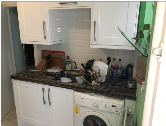
Photo - 86 Kitchen fittings.
