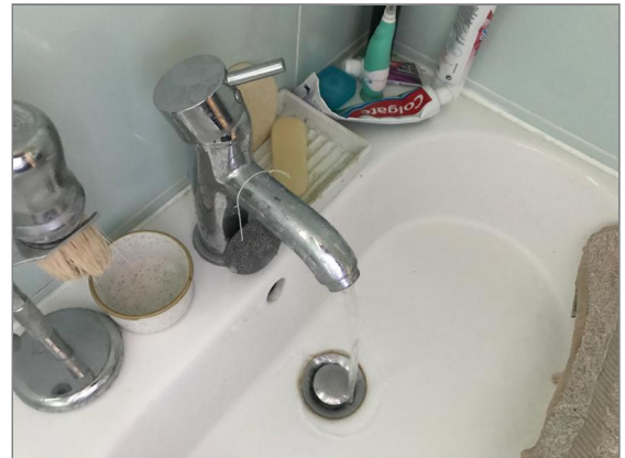
Photo - 107 Testing cold water supply with two outlets open.
