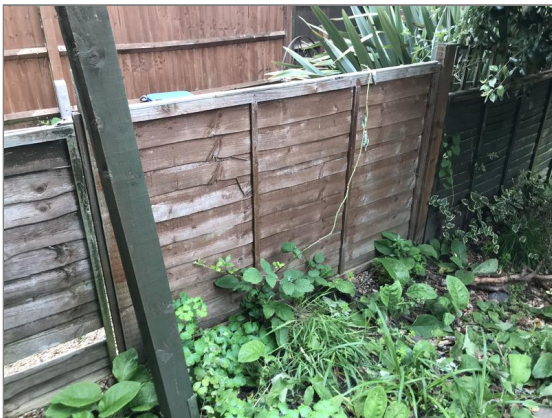
Photo - 126 Fence in rear garden.
