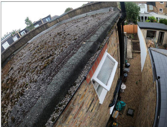
Photo - 17 Felt roof coverings above first floor extension.
