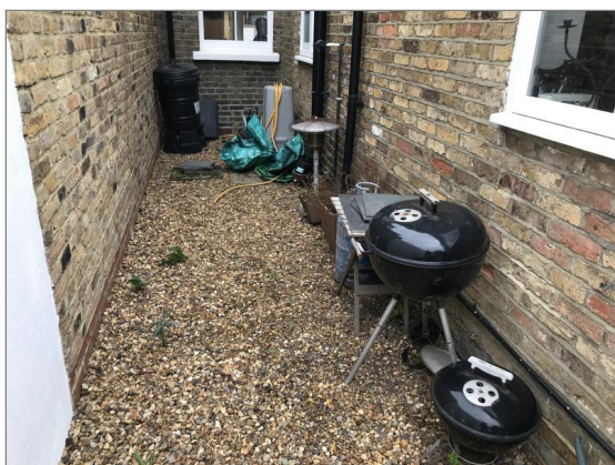
Photo - 180 Inspection chamber located in the rear passageway.
