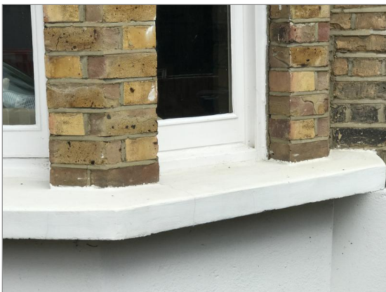
Photo - 70 Decorations of stone window sills.
