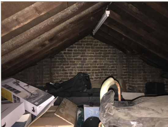
Photo - 72 Main loft void.
