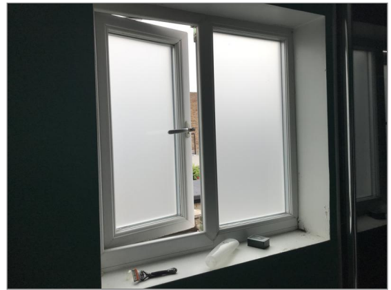
Photo - 52 Bathroom window.
