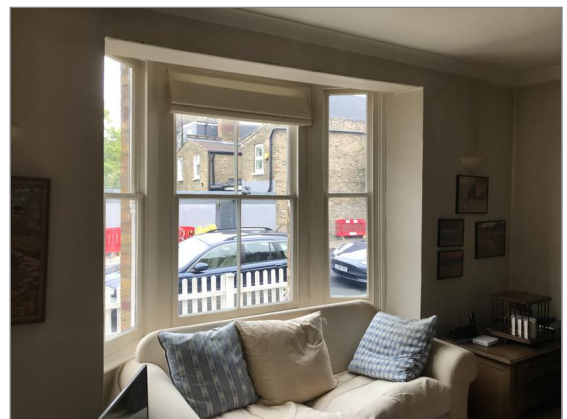
Photo - 110 Front sitting room walls.
