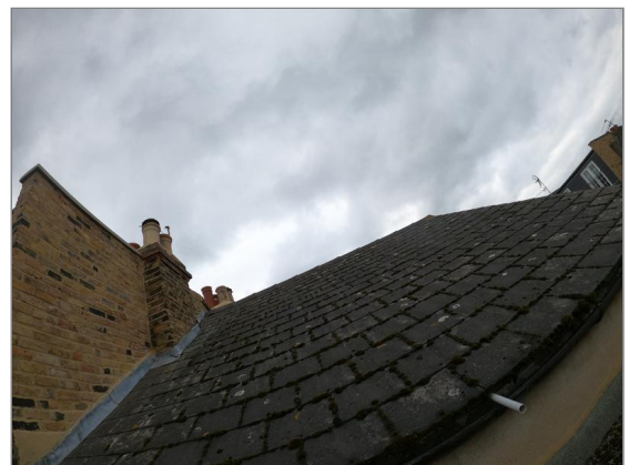
Photo - 14 Rear pitched roof.
