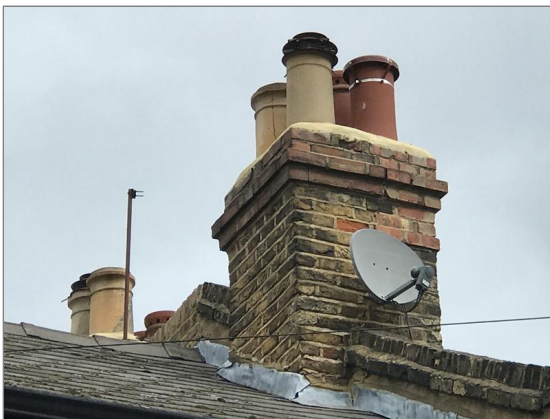
Photo - 6 Front chimney stack.
