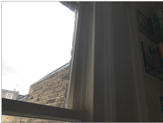
Photo - 57 Counter-weight mechanism removed from rear living room window.
