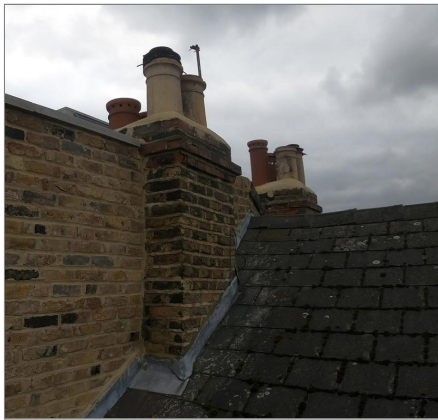
Photo - 8 Elevation view of rear chimney stack.
