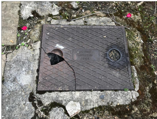
Photo - 176 Crack to inspection chamber lid.
