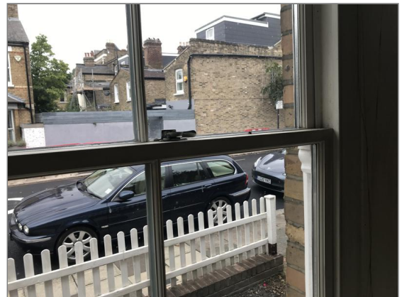
Photo - 54 Counter-weight mechanism removed from living room window.
