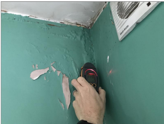
Photo - 119 Damp meter testing to bathroom walls.
