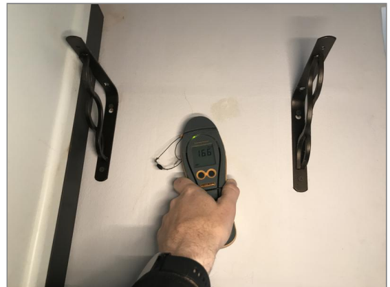
Photo - 102 Damp meter testing to kitchen walls.
