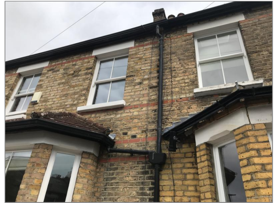
Photo - 21 Rainwater downpipe at the front of the property.
