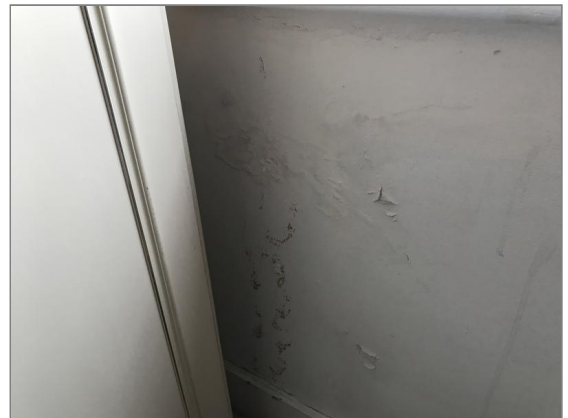
Photo - 126 Front bedroom walls.
