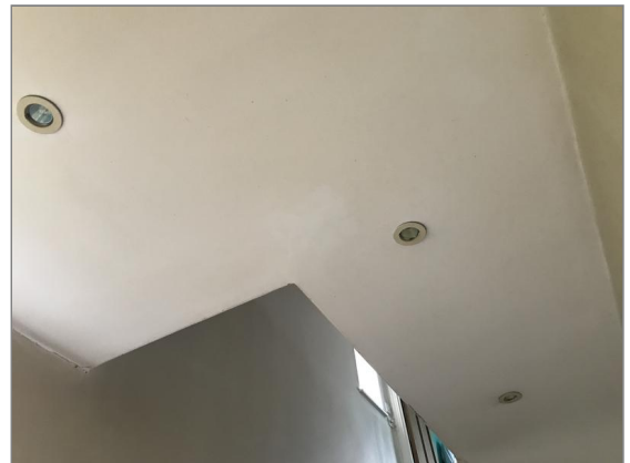
Photo - 91 Ground floor hallway ceiling.
