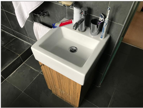
Photo - 158 Basin fittings.
