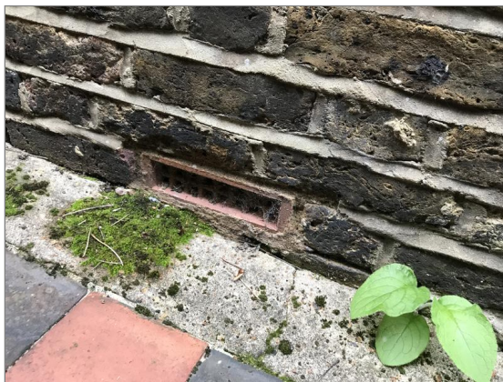
Photo - 133 Sub floor vent close to ground.
