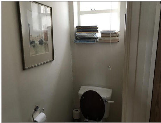
Photo - 123 WC walls.
