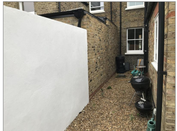
Photo - 41 Extension built astride the boundary.
