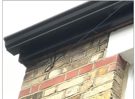
Photo - 69 uPVC fascias at the front of the property.
