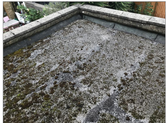
Photo - 18 Felt roof coverings above ground floor extension.
