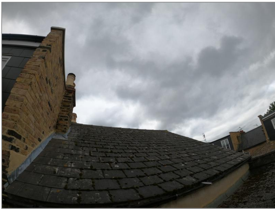
Photo - 15 Raised parapet wall to side of rear pitched roof.
