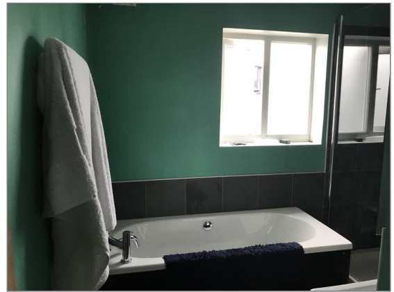
Photo - 118 Bathroom walls.
