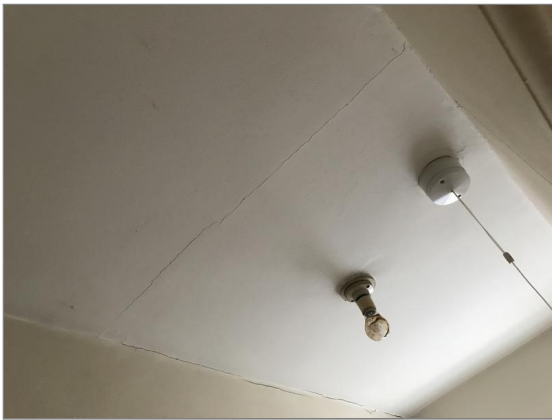
Photo - 88 WC ceiling.
