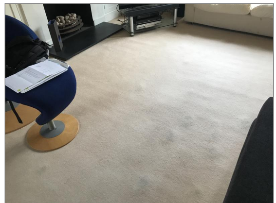
Photo - 136 Floorboards visible through living room floor.
