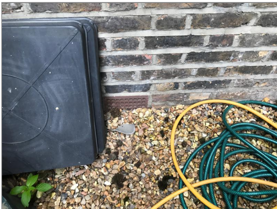
Photo - 40 Sub floor vent to back of the property.
