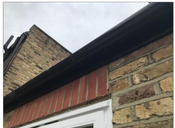
Photo - 71 Timber fascias at the rear of the property.
