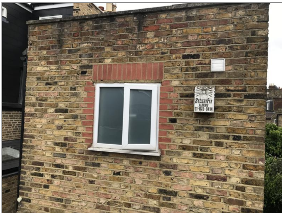
Photo - 34 Rear bathroom walls.
