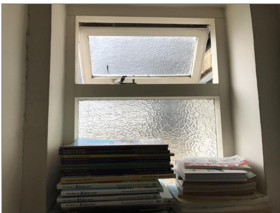
Photo - 49 WC window.
