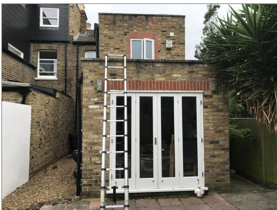
Photo - 42 Rear elevation of the building.
