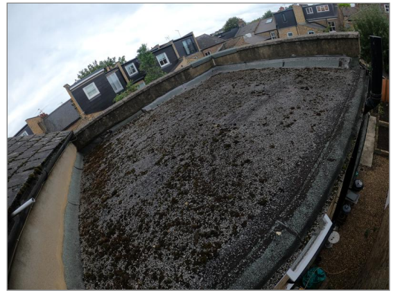
Photo - 16 Felt roof coverings above first floor extension.
