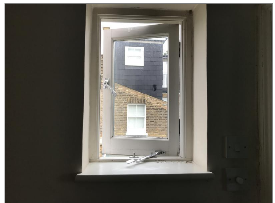
Photo - 50 Landing window.
