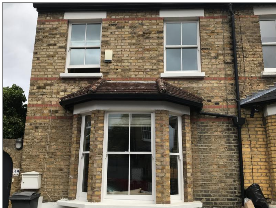
Photo - 43 Double glazed windows at front elevation of the property.
