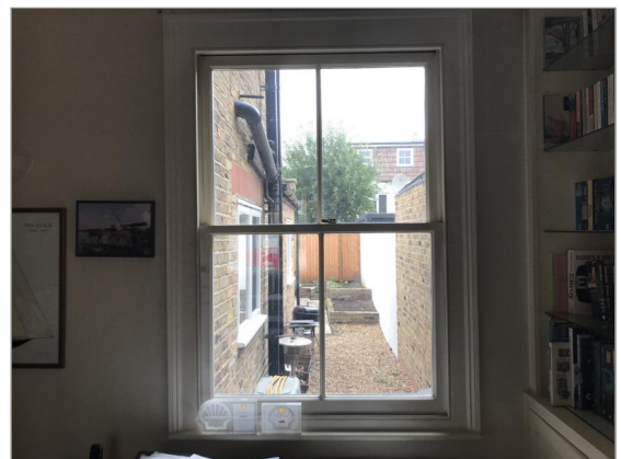
Photo - 56 Rear living room window.
