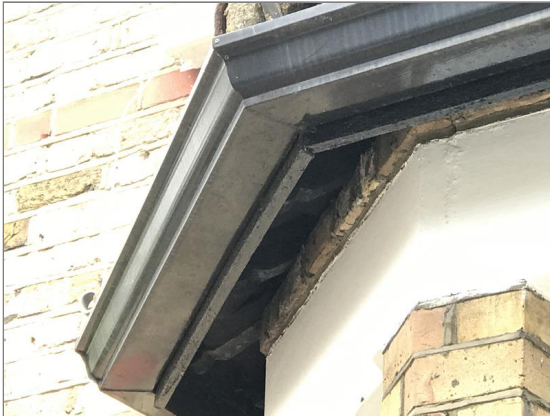
Photo - 68 Timber fascias at front of the property.
