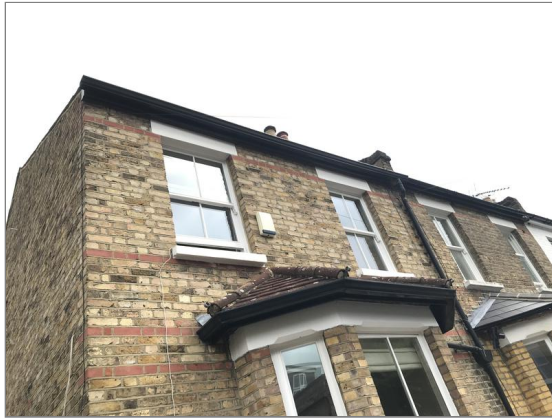
Photo - 20 Rainwater guttering at the front of the property.
