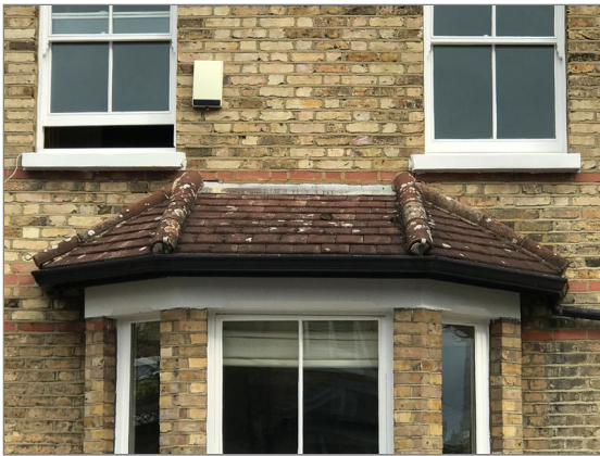
Photo - 9 Plain tiles to bay roof.
