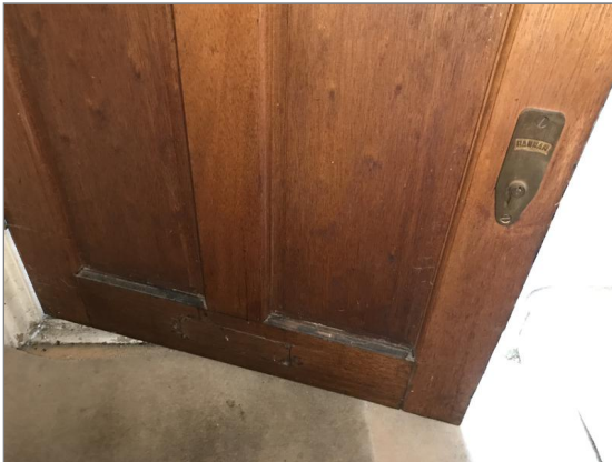
Photo - 64 Internal face of front door.
