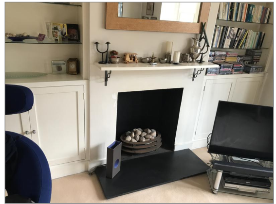
Photo - 142 Living area gas fire.
