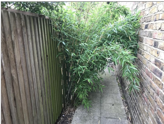
Photo - 190 Mature bamboo growth at the side of the property.
