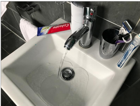
Photo - 169 Testing cold water supply.
