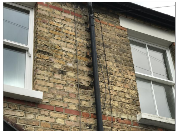
Photo - 29 Repaired brickwork to the front elevation.
