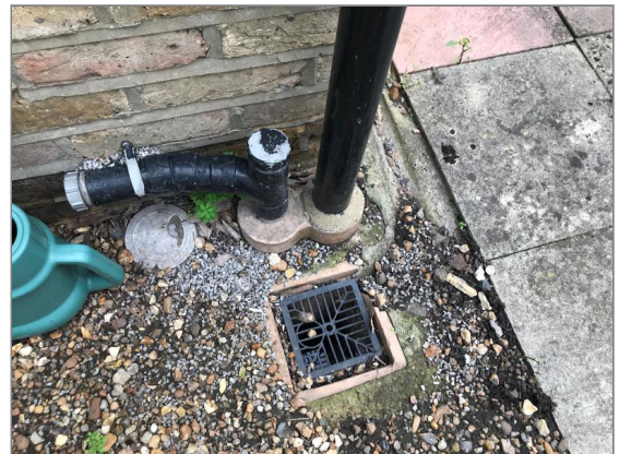
Photo - 27 Back inlet gully at the back of rear addition.
