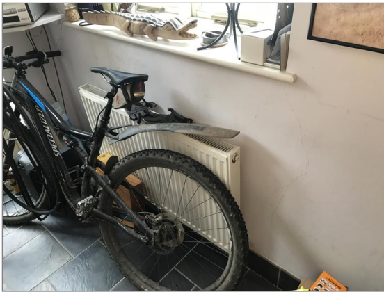
Photo - 99 Cracking to dining area walls.
