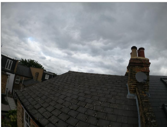
Photo - 13 Elevated view of front pitched roof.
