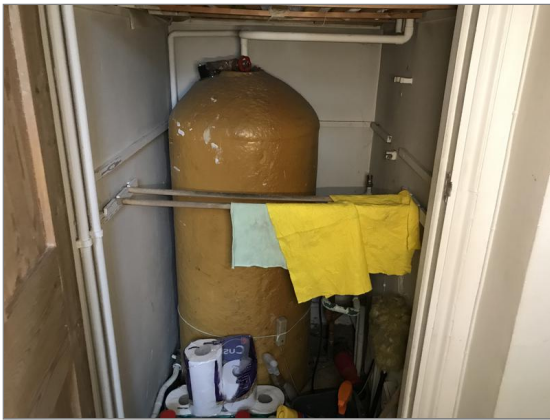
Photo - 173 Hot water cylinder
