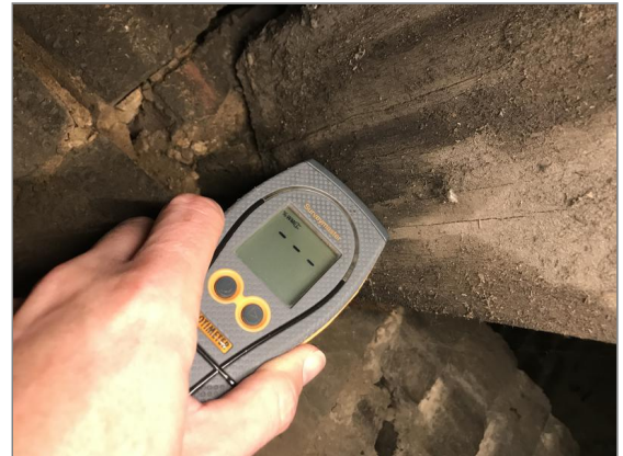
Photo - 77 Damp meter testing to roof timbers.
