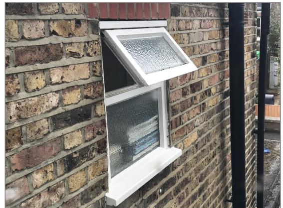
Photo - 48 WC window.
