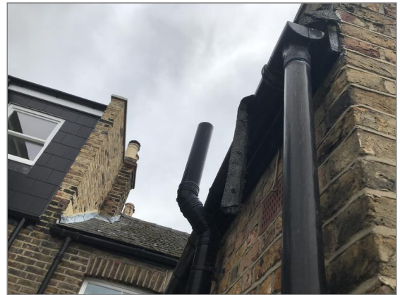
Photo - 23 Rainwater goods at the rear of the property.
