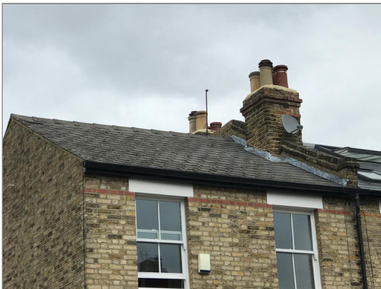
Photo - 11 Front pitched roof covering.
