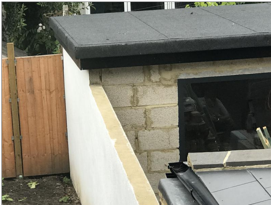
Photo - 195 Roof structure oversailing boundary wall.
