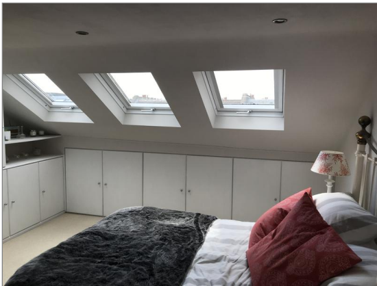
Photo - 150 Larger second floor bedroom walls
