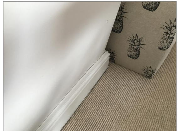
Photo - 151 Larger second floor bedroom walls
