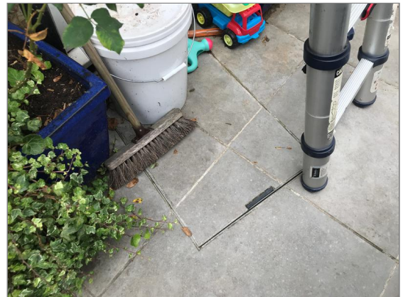
Photo - 219 Inspection chamber in rear garden
