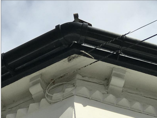
Photo - 73 Timber fascias and soffits
