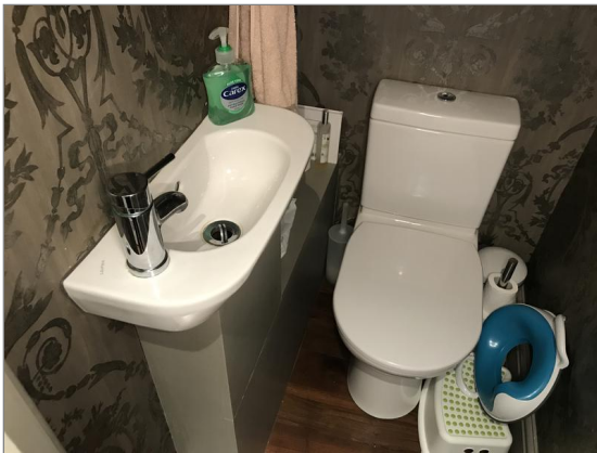
Photo - 200 Ground floor WC fittings
