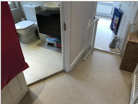
Photo - 158 Rear second floor bedroom floors
