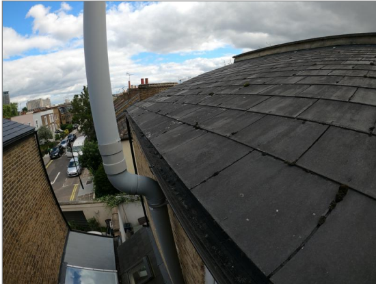
Photo - 27 Rainwater guttering to rear outrigger roof
