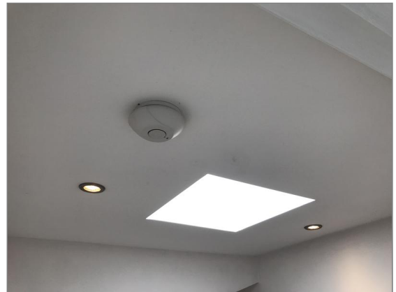
Photo - 81 Second floor landing ceiling
