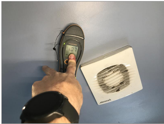
Photo - 86 Damp meter testing to second floor bathroom ceiling
