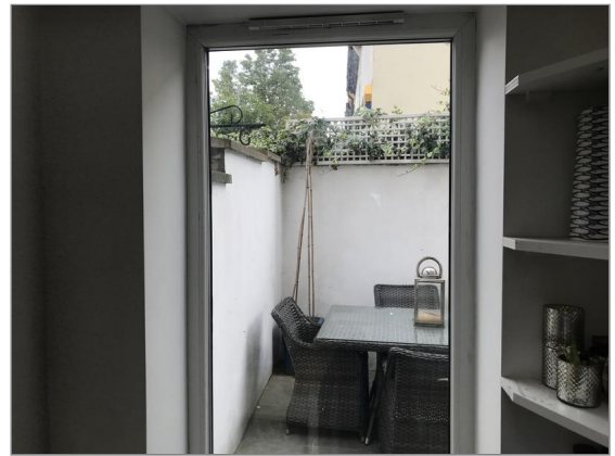
Photo - 59 Fixed glazing pane at rear of side addition
