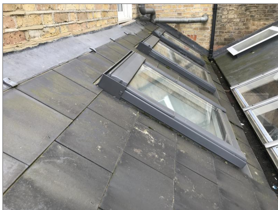
Photo - 21 Side addition roof
