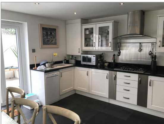
Photo - 118 Kitchen walls
