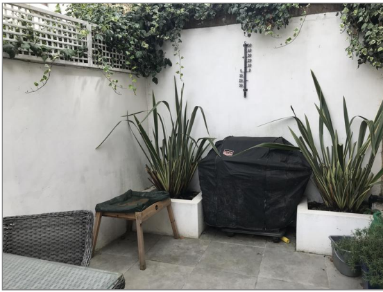
Photo - 229 Walls in rear garden
