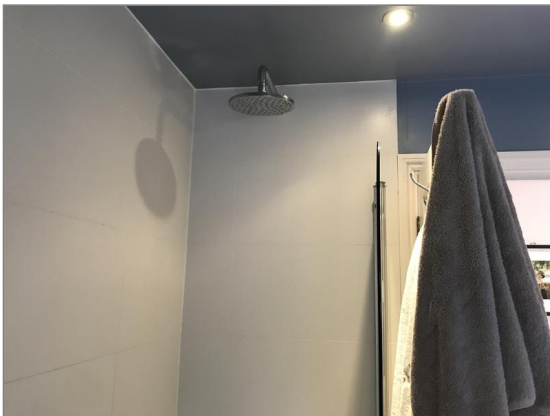
Photo - 192 Second floor bathroom fittings
