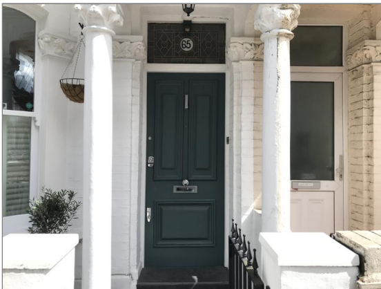
Photo - 60 Front door
