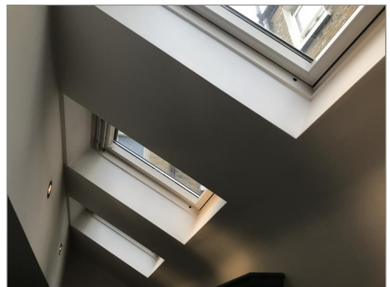
Photo - 103 Side addition ceiling
