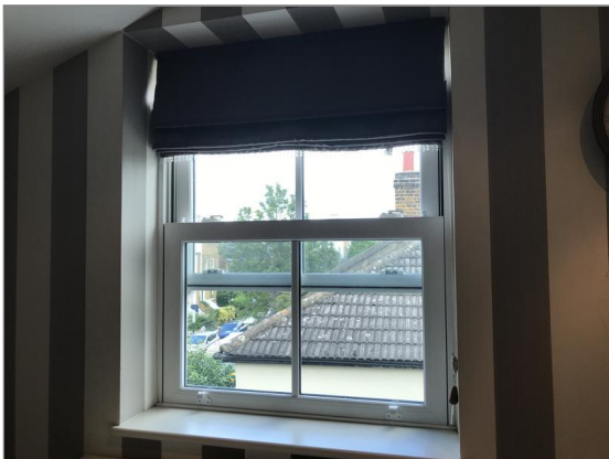
Photo - 48 Rear second floor bedroom window
