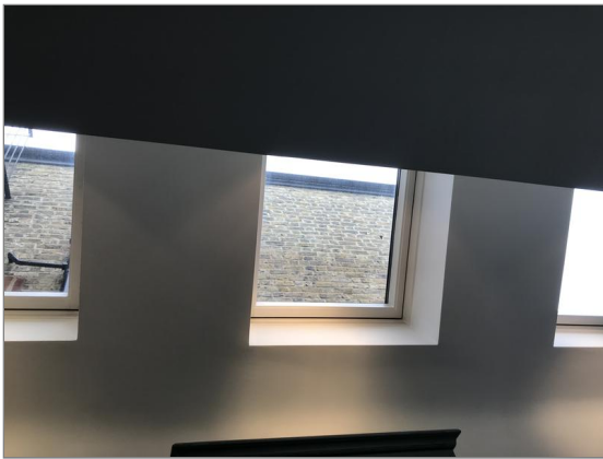
Photo - 58 Side addition windows
