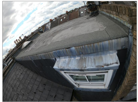
Photo - 18 Rear elevation of flat mansard roof
