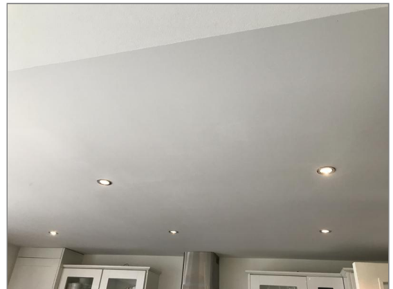
Photo - 101 Kitchen ceiling
