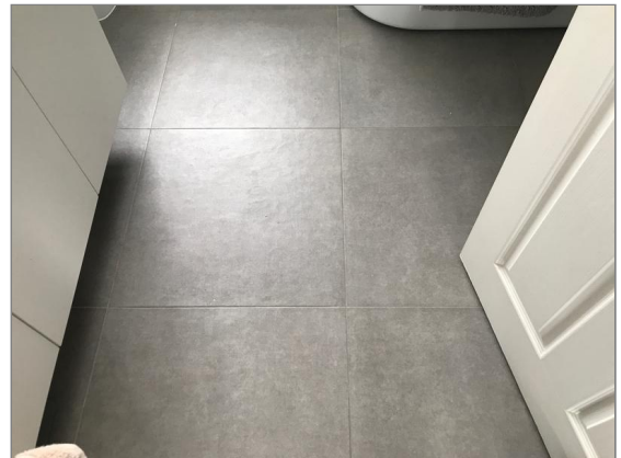
Photo - 157 Ceramic floor tiles to master en-suite
