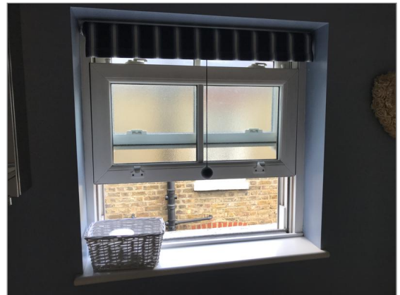
Photo - 47 Second floor bathroom window
