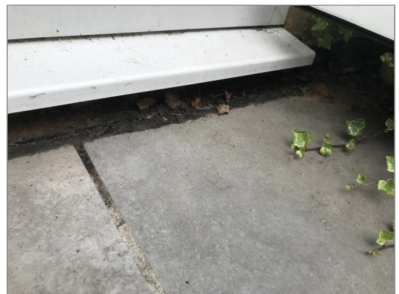
Photo - 228 Channel drain in rear garden
