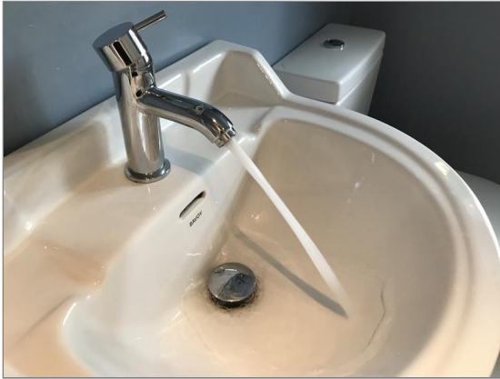
Photo - 210 Testing cold water supply with one outlet open
