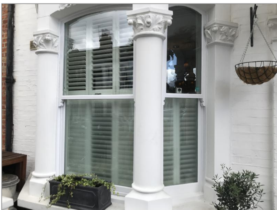
Photo - 56 Front sitting room windows
