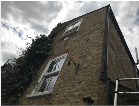
Photo - 40 Rear elevation of building
