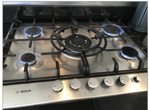
Photo - 209 Testing gas supply to hob
