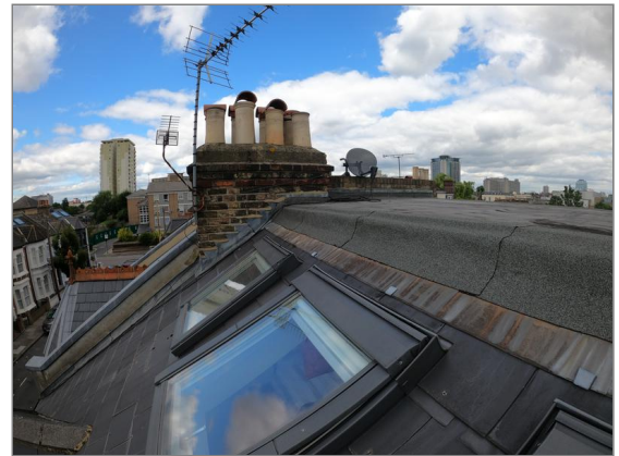
Photo - 12 Elevated view of main chimney stack
