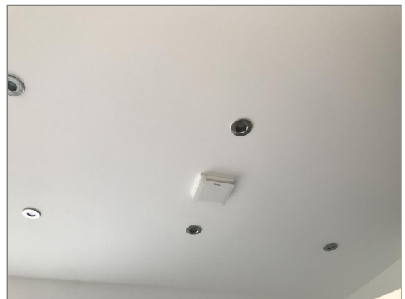
Photo - 91 First floor master en-suite ceiling
