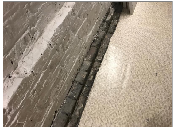
Photo - 202 Exposed brickwork walls in basement
