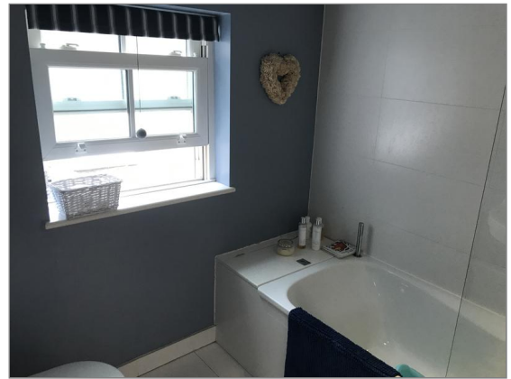
Photo - 145 Second floor bathroom walls
