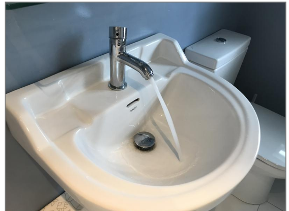
Photo - 216 Testing hot water supply with two outlets open
