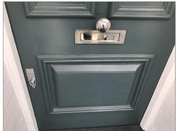
Photo - 61 Slight tarnish to front door fittings
