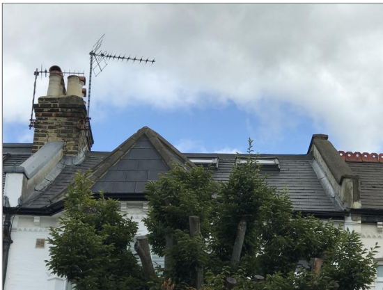
Photo - 13 Front pitched roof
