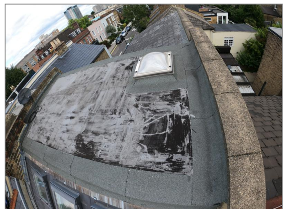
Photo - 16 Elevated view of flat mansard roof
