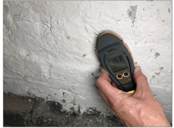
Photo - 204 Damp meter testing to walls in basement
