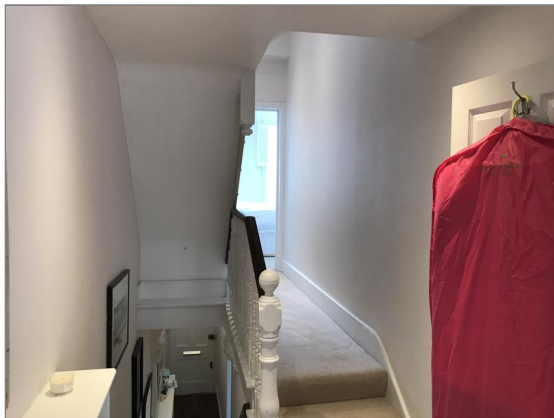
Photo - 128 First floor landing walls
