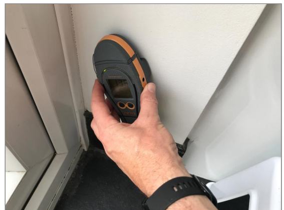
Photo - 119 Damp meter testing to kitchen walls
