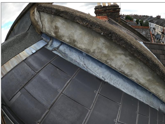
Photo - 15 Lead flashings at side of front pitched roof
