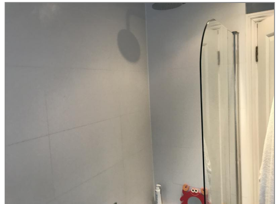
Photo - 147 Tiling within second floor bathroom
