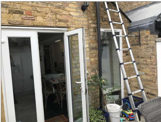
Photo - 42 Walls to side addition
