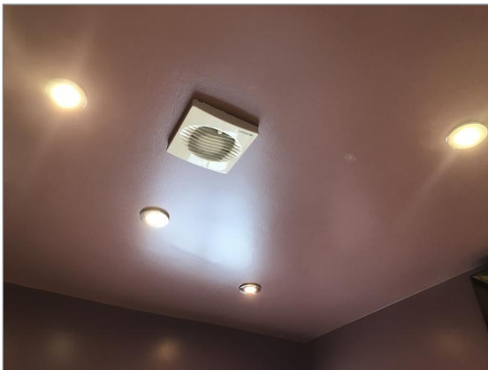
Photo - 94 First floor bathroom ceiling
