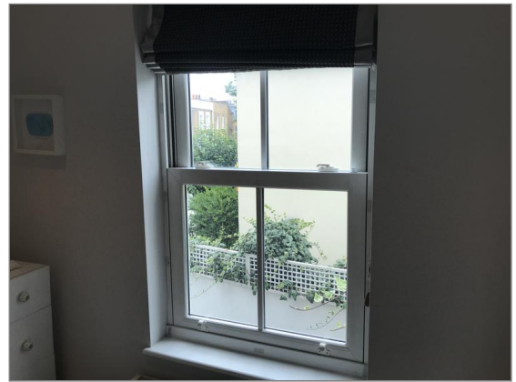
Photo - 53 Rear first floor bedroom window
