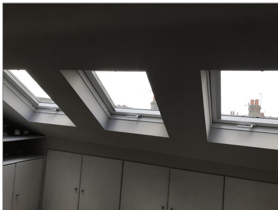
Photo - 44 Larger second floor bedroom windows
