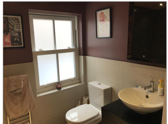
Photo - 129 First floor bathroom walls
