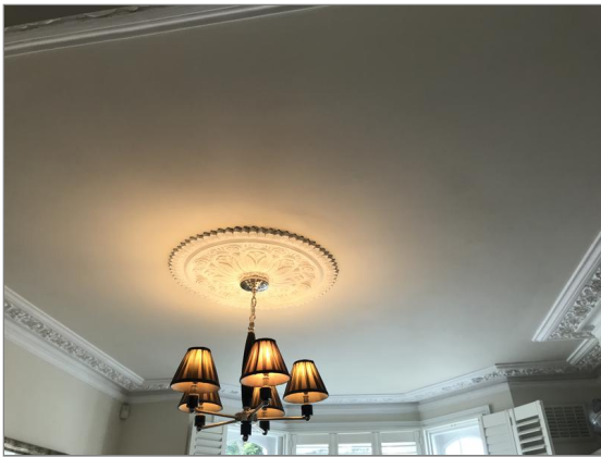
Photo - 98 Front sitting room ceiling
