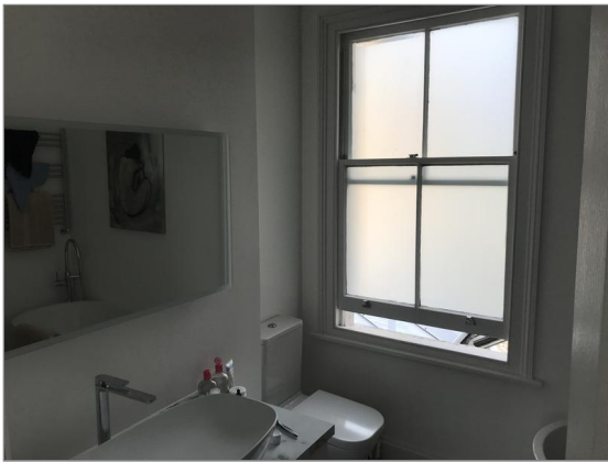
Photo - 138 Master en-suite walls
