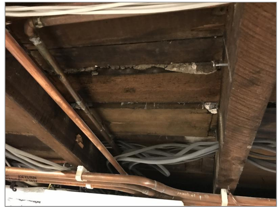
Photo - 163 Suspended timber floor at ground floor level
