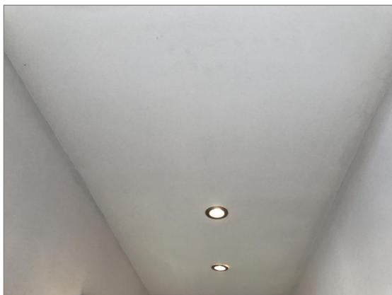
Photo - 84 Second floor landing ceiling
