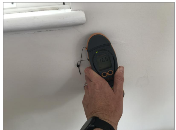
Photo - 149 Damp meter testing to rear second floor bedroom walls
