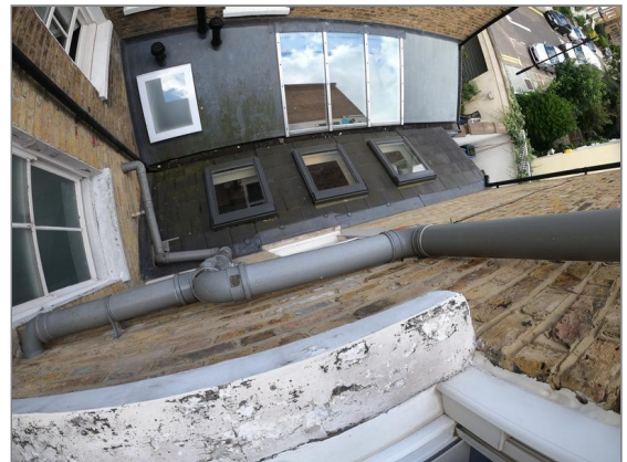
Photo - 20 Side addition roof
