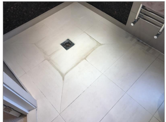
Photo - 159 Tiling to second floor shower room floor
