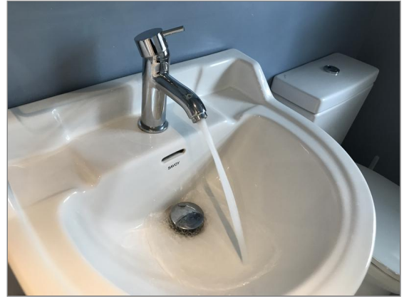
Photo - 211 Testing cold water supply with two outlets open
