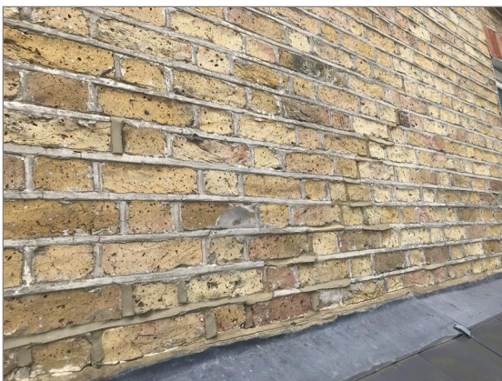
Photo - 38 Repointed brickwork at rear of property
