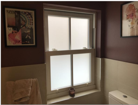
Photo - 52 First floor bathroom window
