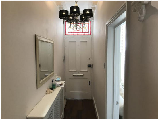
Photo - 104 Entrance hallway walls
