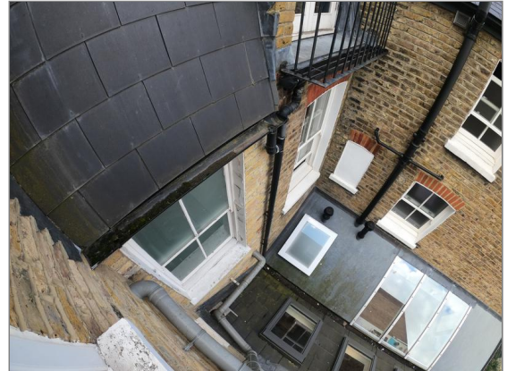
Photo - 28 Rainwater downpipe at rear of mansard
