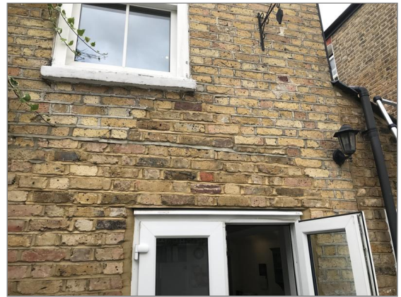
Photo - 41 Cracking repair above kitchen door
