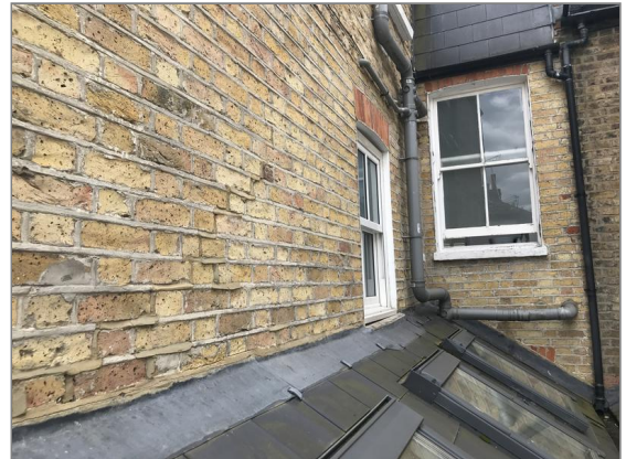
Photo - 37 Cracking repair at rear of property
