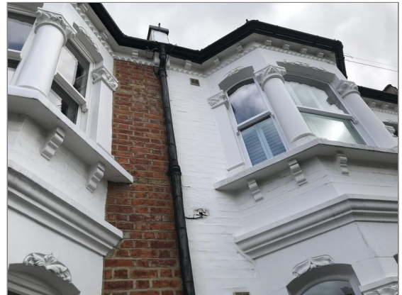
Photo - 24 Cast iron downpipe at front of property
