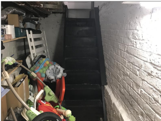
Photo - 201 Stairs leading down to basement
