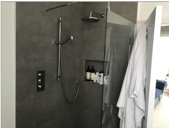
Photo - 140 Tiling to master en-suite shower enclosure
