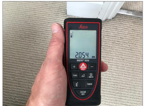
Photo - 83 Height of ceiling at second floor level
