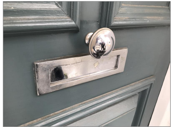
Photo - 63 Front door fittings
