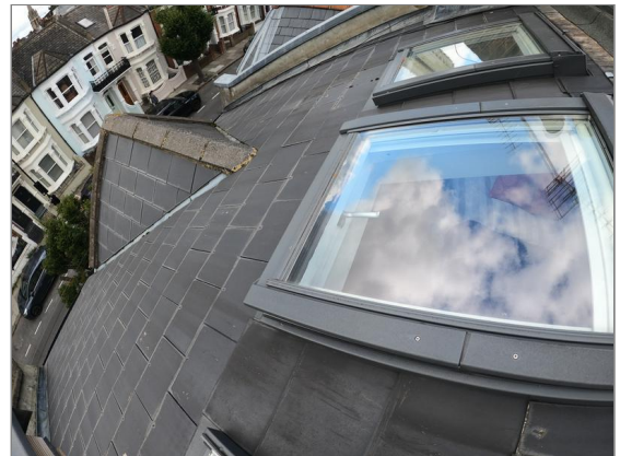
Photo - 14 Elevated view of front pitched roof
