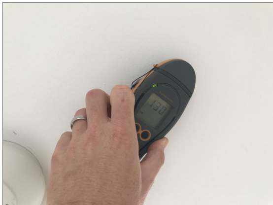
Photo - 82 Damp meter testing to second floor landing ceiling
