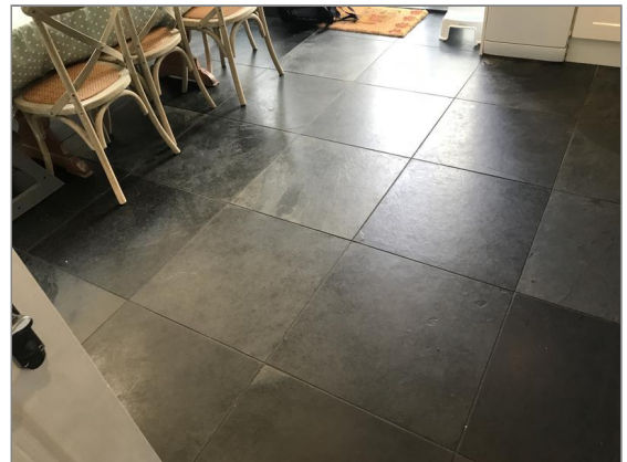
Photo - 165 Tiles to kitchen area
