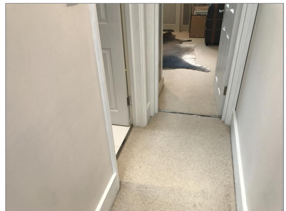
Photo - 153 Lower second floor landing level
