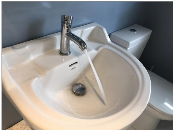
Photo - 215 Testing hot water supply with one outlet open
