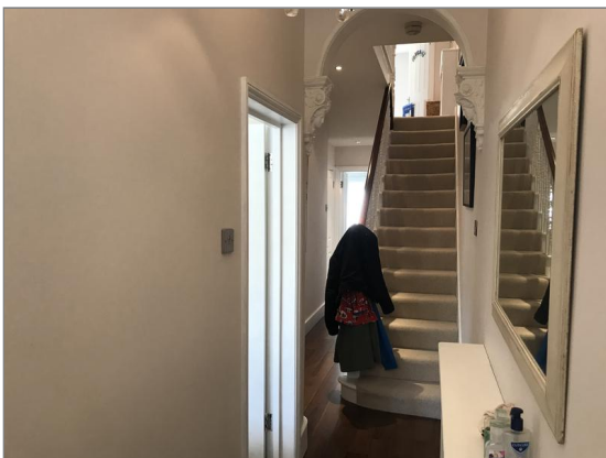
Photo - 106 Entrance hallway walls
