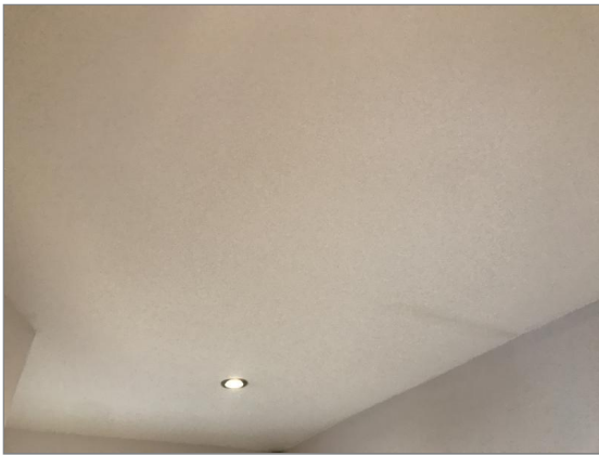
Photo - 92 First floor master changing area ceiling
