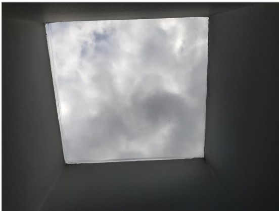
Photo - 46 Roof light above second floor landing
