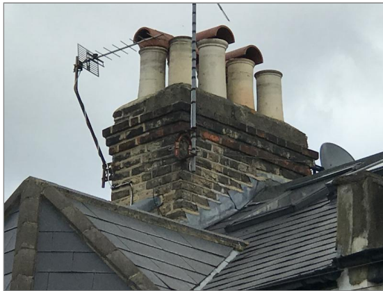
Photo - 11 Main stack
