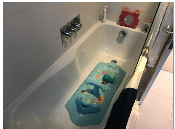
Photo - 191 Second floor bathroom fittings
