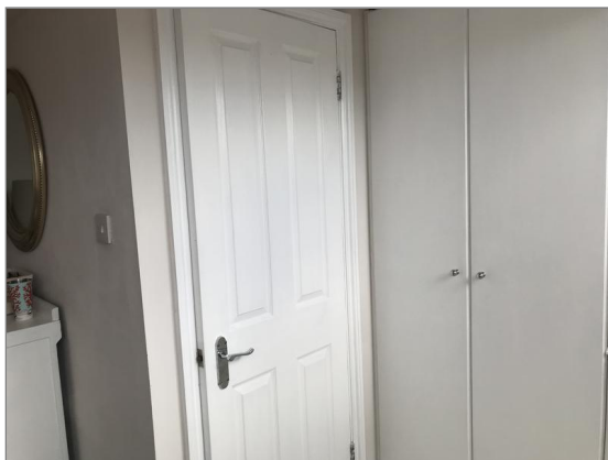
Photo - 183 Bedroom door at second floor level
