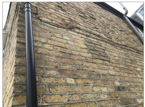
Photo - 39 Brickwork at rear of property
