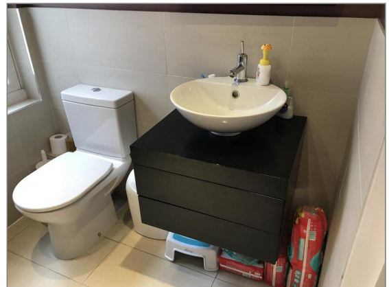
Photo - 197 First floor shower room fittings
