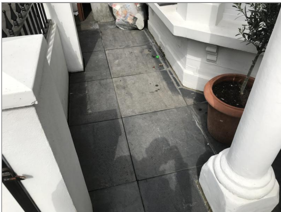
Photo - 225 Paving in front garden
