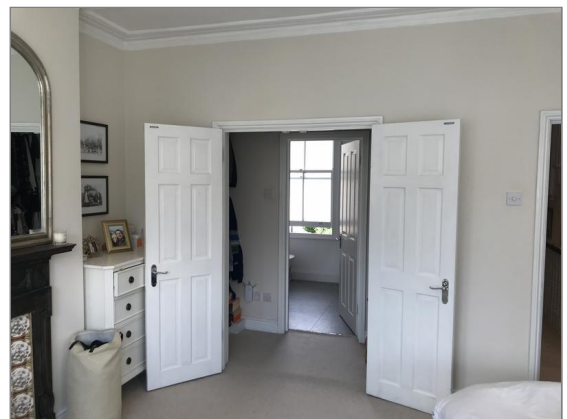
Photo - 137 Master bedroom walls
