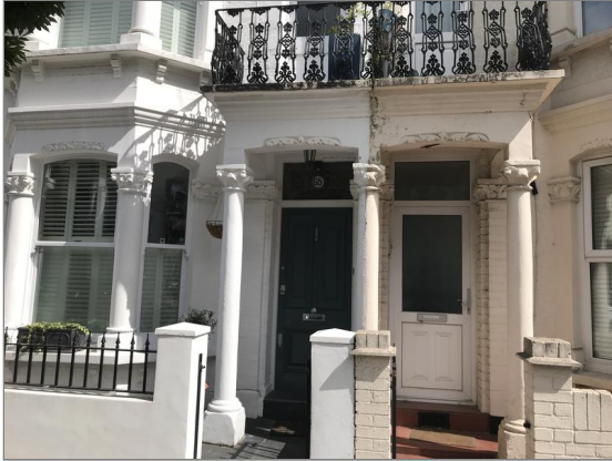
Photo - 68 Porch structure
