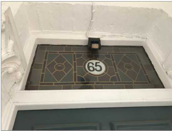
Photo - 62 Leaded overhead light
