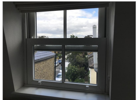
Photo - 45 Sash window to rear of larger second floor bedroom
